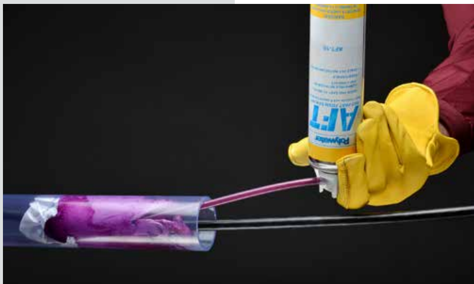
Installation of Polywater AFT-16
